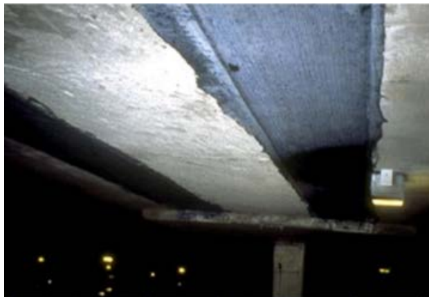
Figure 2-9 - FRP strips added to bottom of flexural beams [39]
