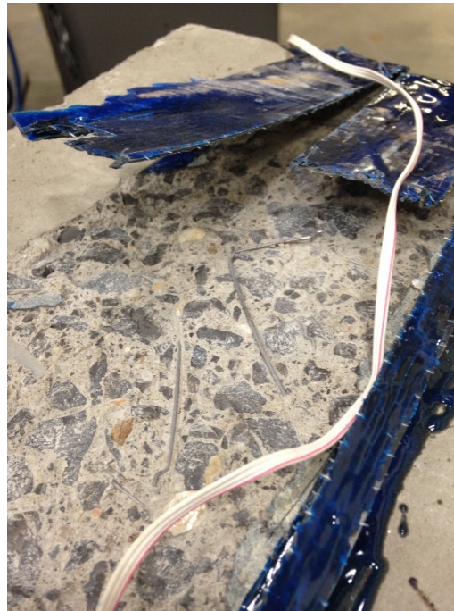
Figure 1-7 - Exposed Aggregate of SFRC Panels
