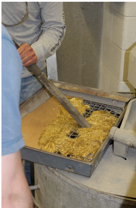
Figure 1-5 - Adding steel fibres to the UHPFRC mix
