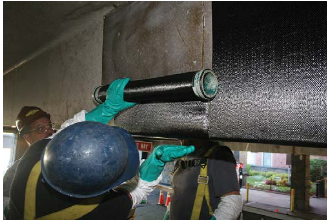
Figure 2-8 – FRP wet lay-up on concrete beam [38]
