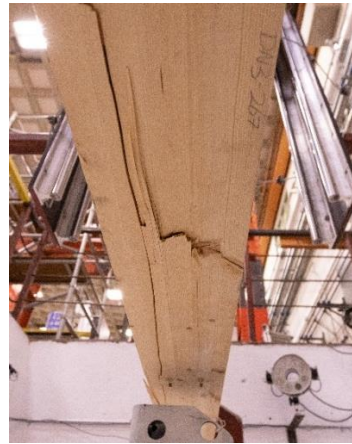
(c) Underside of specimen after failure
