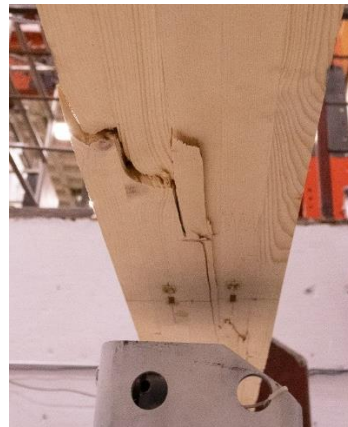
(c) Underside of specimen after failure
