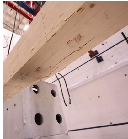
(c) Underside of specimen after failure
