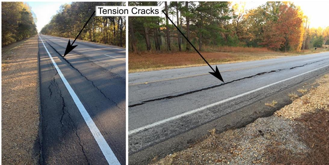
Figure 23 Road Damage Caused by Expansive Soil (Coating Industry News, 2016)
